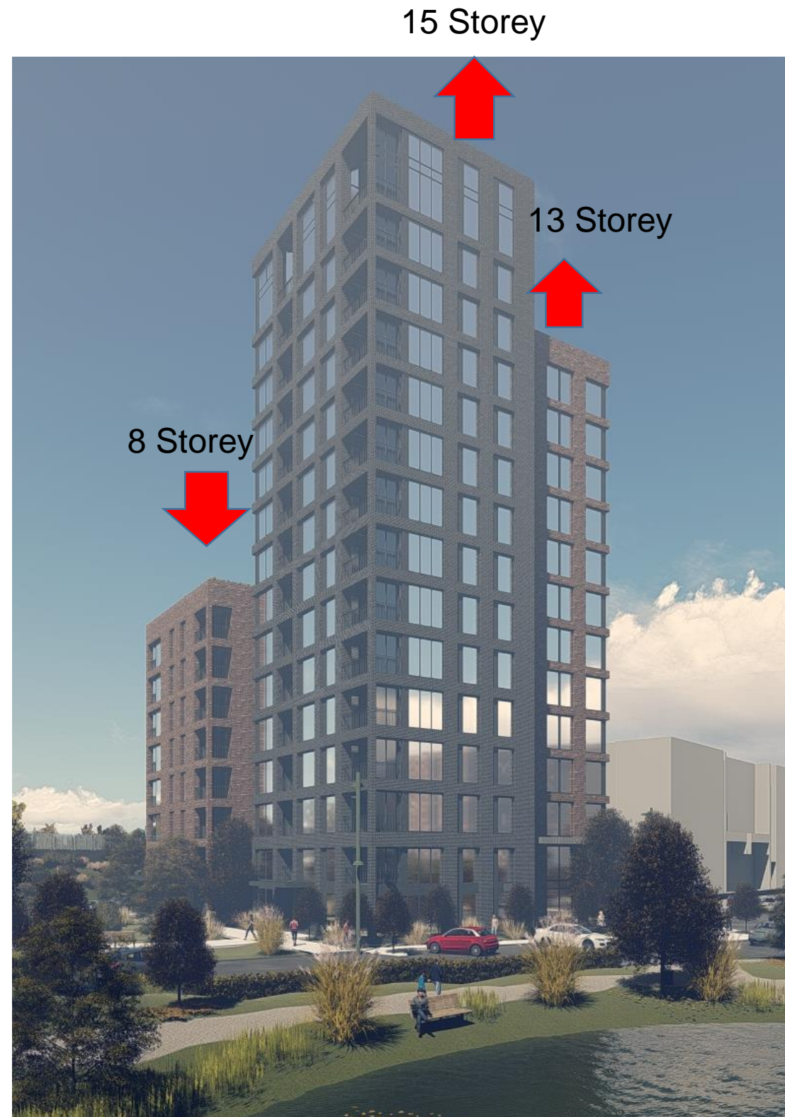
View from the West
