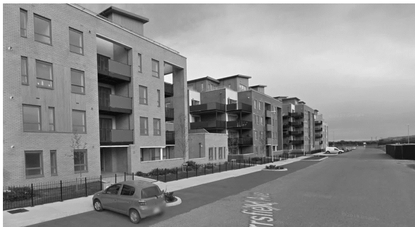
View eastward of existing apartments on north side of Marrisfield Avenue
